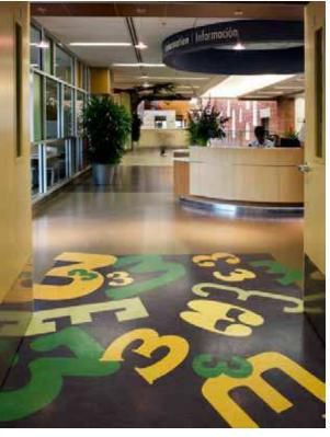
Intertech Flooring installed more than 50 different flooring products on the Dell Children's project. Green-friendly products included natural linoleum with low- or no-VOC adhesives, raised access flooring with underfloor air, and carpeting made with recycled content.
