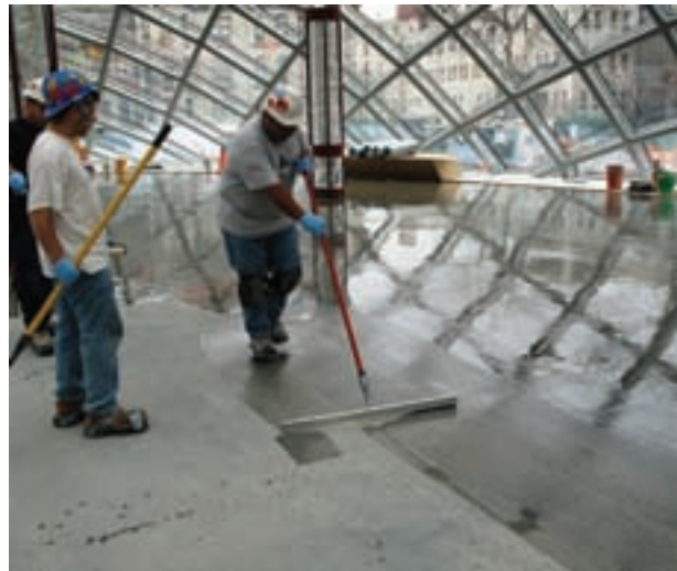
Today's professional flooring contractor has more options than ever to help it resolve potential moisture related problems such as Mapei's Planiseal, which is designed to treat concrete slabs of at least 14 days that exhibit certain moisture vapor emission rates.
